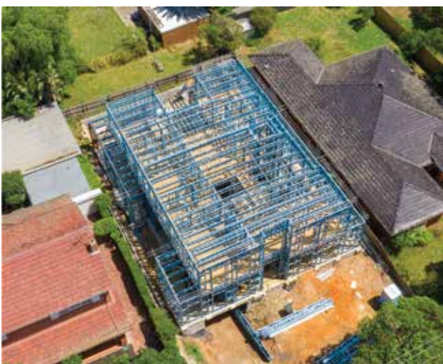
Tourello Ave, Hawthorn East
